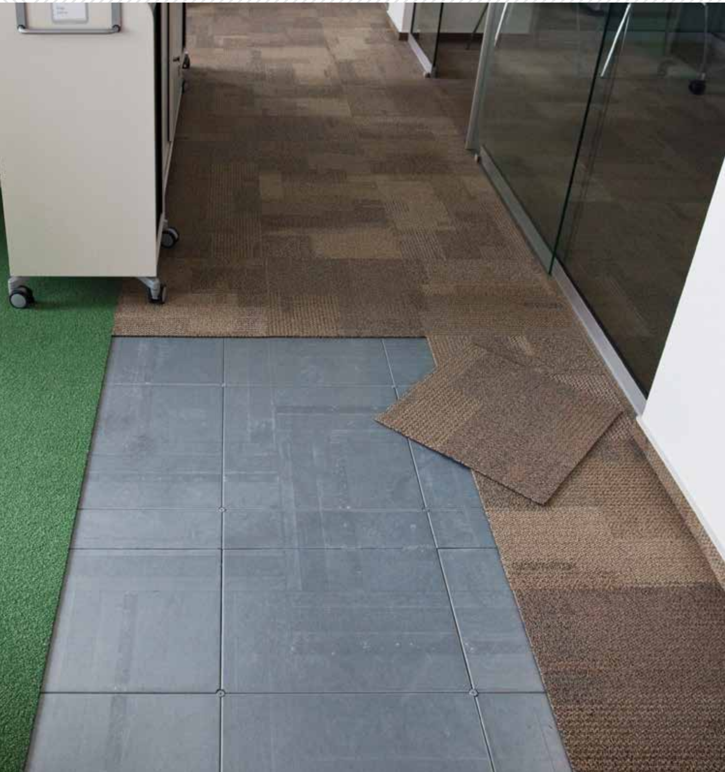
Standard Intercell installation with carpet tiles
